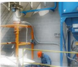
In a food production plant has been installed a recovery of the starch. Sucked into a filter, the starch is presented as fine dust particles, that had to be put in a big bag to be stored in a designated area.
